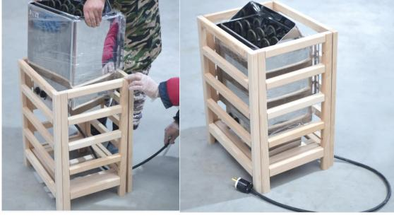
5. Install the vertical bench (note: pull the stove plug line through the dent under vertical bench and connect it .
